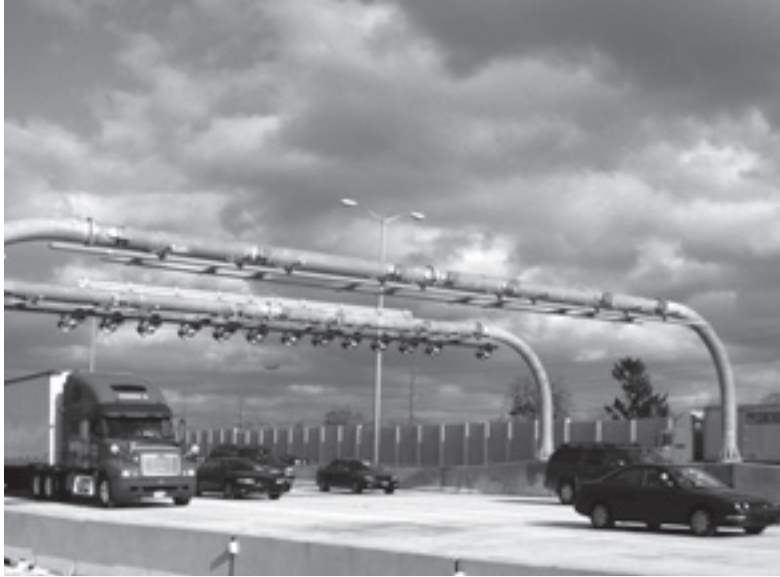
Open road tolling lanes at the Irving Park Road Toll Plaza on the Tri-State Tollway (I-294) in Illinois.
